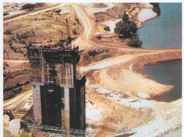
Construction of the Ord River Dam intake tower
